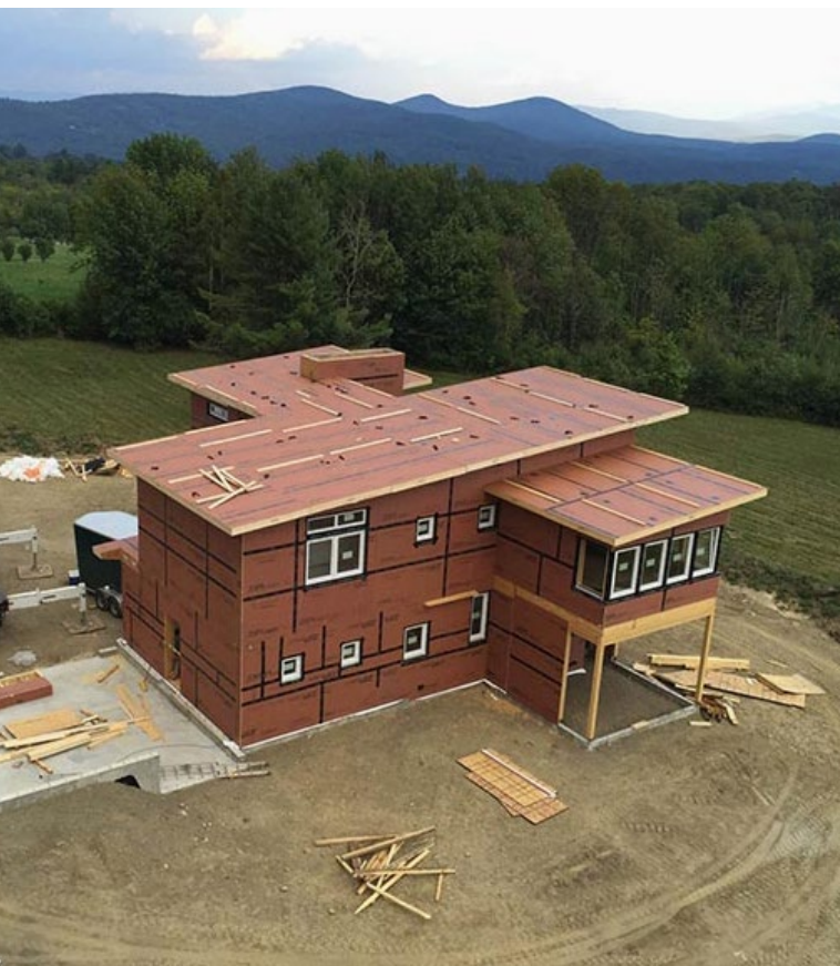
Fig. 1 / 3 Mountain Modern in the building phase.
